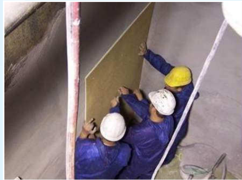
Reconstruction with Composite-panels
